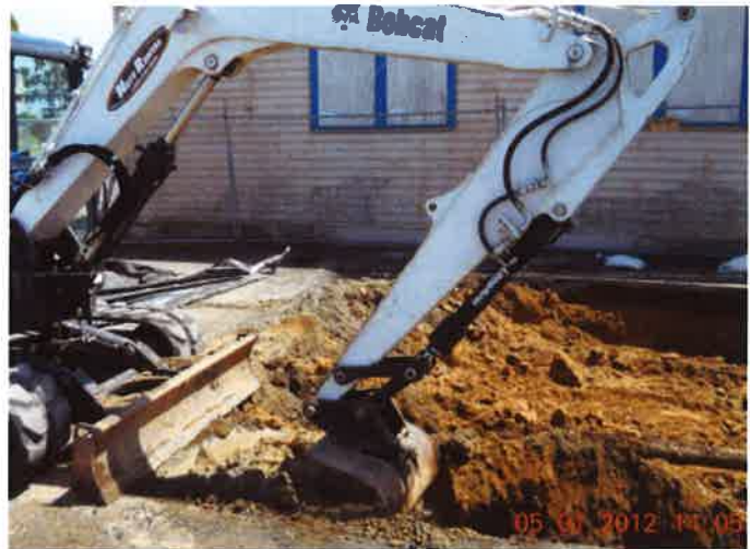
Excavation at Site 33
