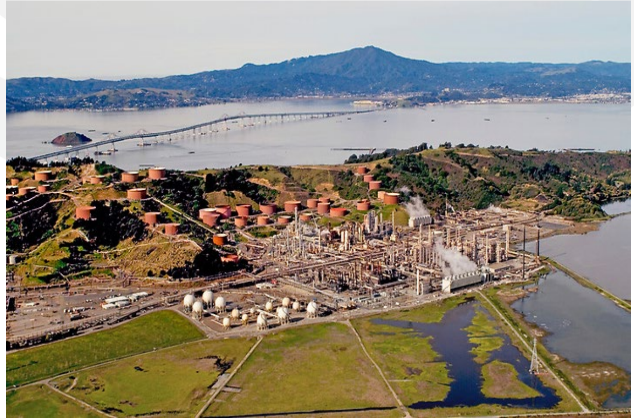
Chevron Richmond Refinery
