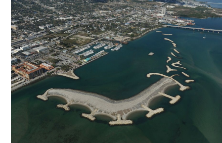
New Island Construction
