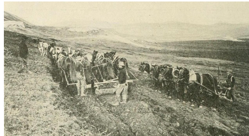
Miocene Ditch construction, Nome River, AK, 1901-03
