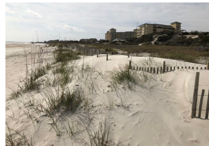
Beach and Dune Construction
