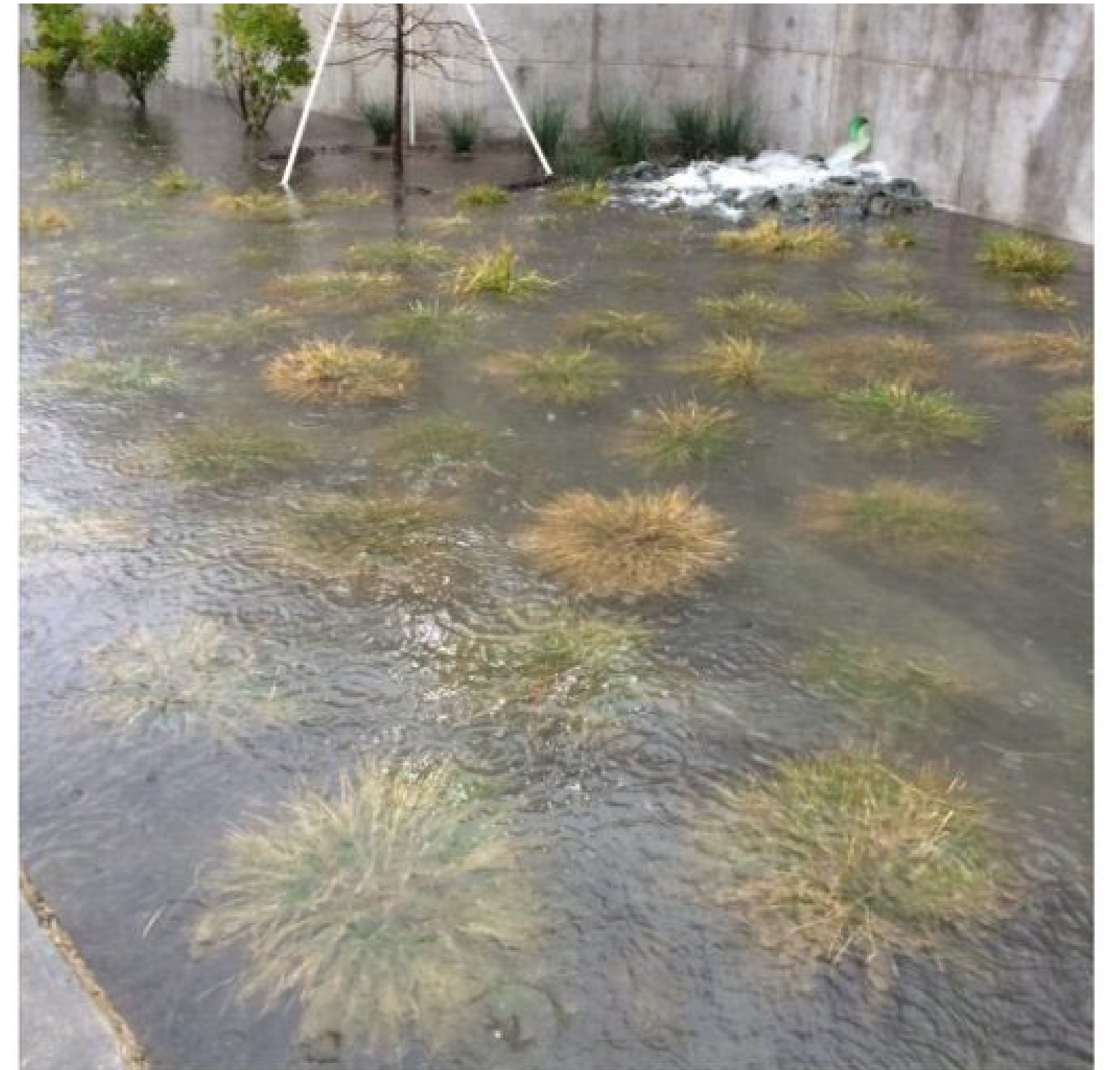
Green infrastructure cell flooding during a rain event at El Cerrito High School, California
