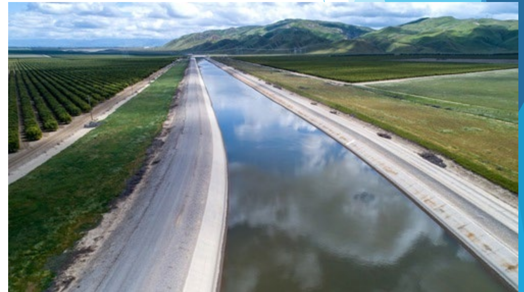
DWR Photo of California Aqueduct
