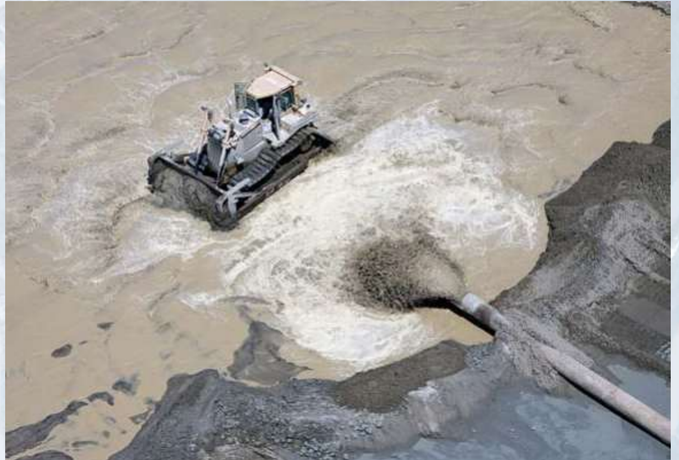
Hamilton Wetlands Restoration
