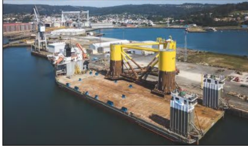
2) Loadout onto semi sub
