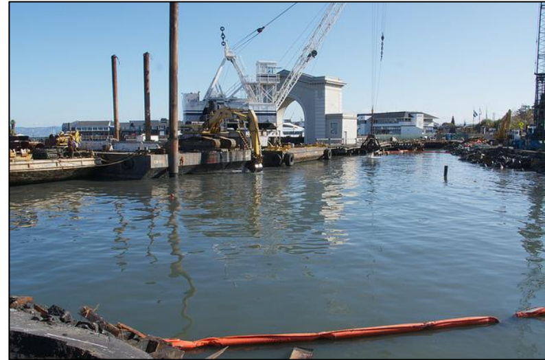
Photo: Pier 43-12 Sea Wall Repairs 11-2011 by Dave R
