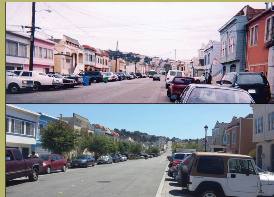
Newcomb Street before and after the low impact development project curbing flooding. Photos by San Francisco Planning Department (top) and James Muller (bottom).
