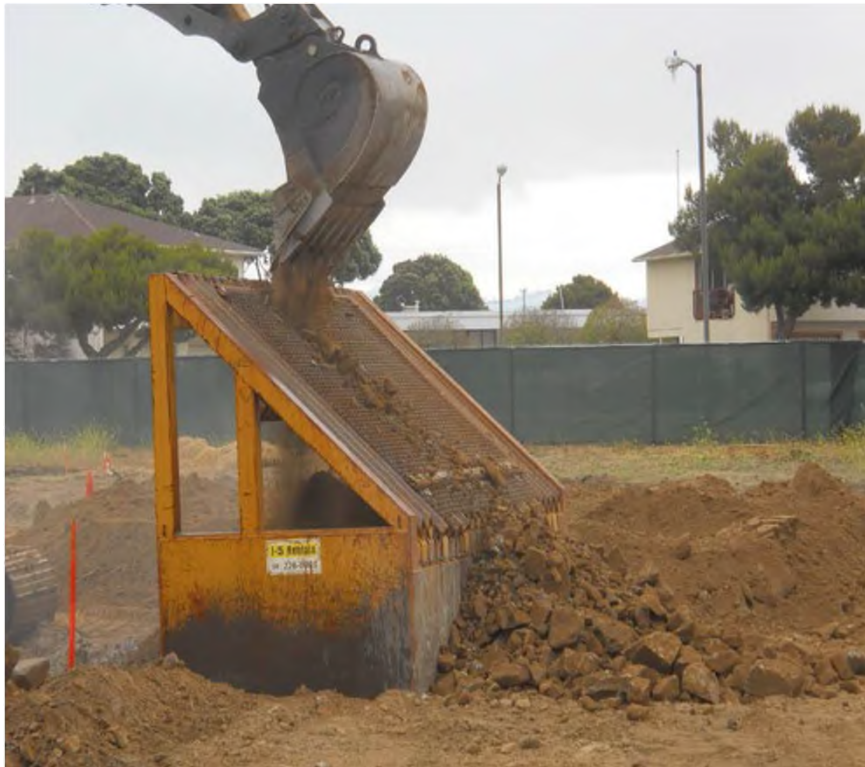
Screening rock from soil in the excavation areas
