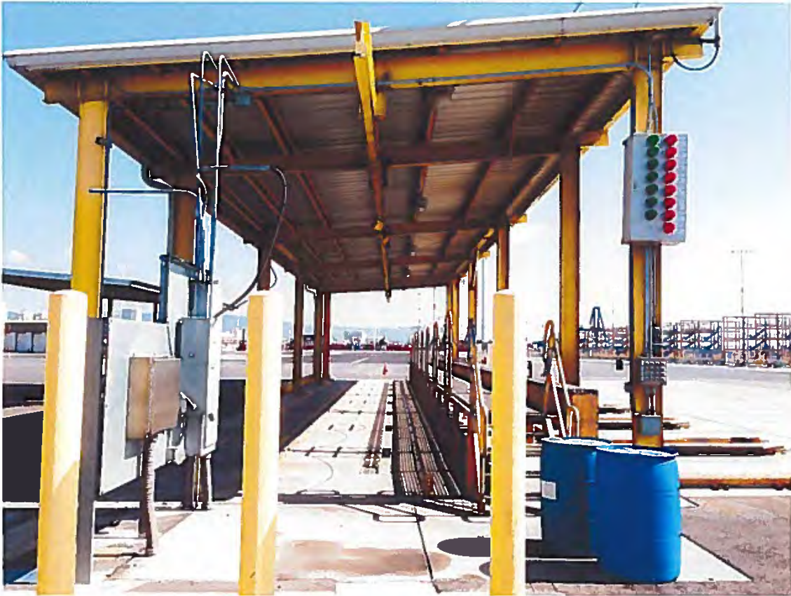
End View of Reefer Wash Rack
