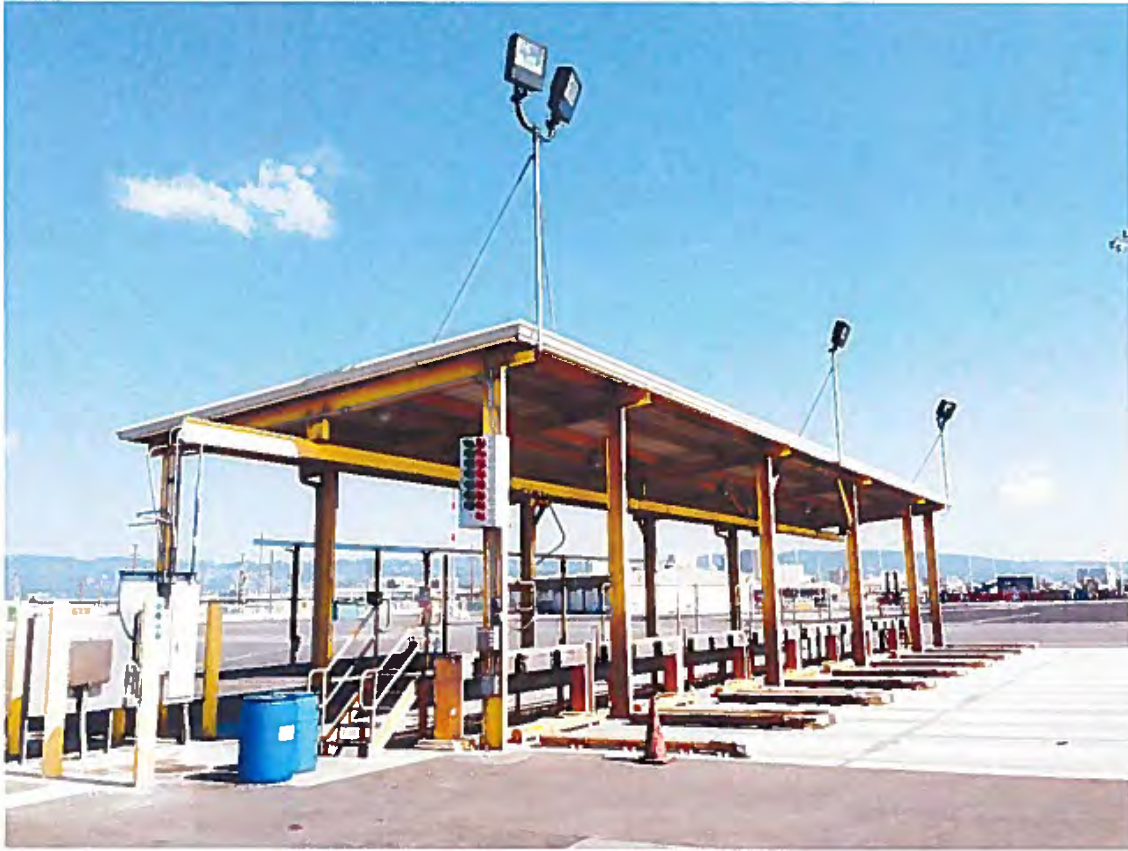
Reeper Wash Rack structures and associated equipment
