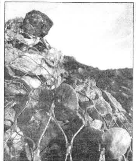
As part of the Living Shorelines project, scientists placed mesh bags full of oyster shells (pictured at distance on the left and in closeup on the right) off of the San Rafael coast.
