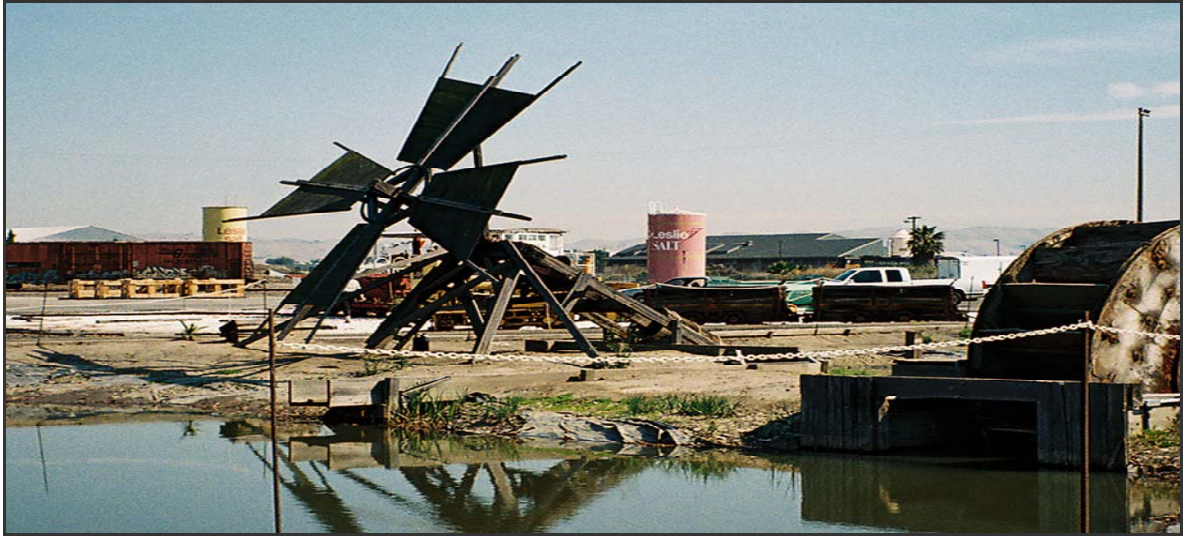
Figure 11: Archimedes Screw Pump (Photo by author)
