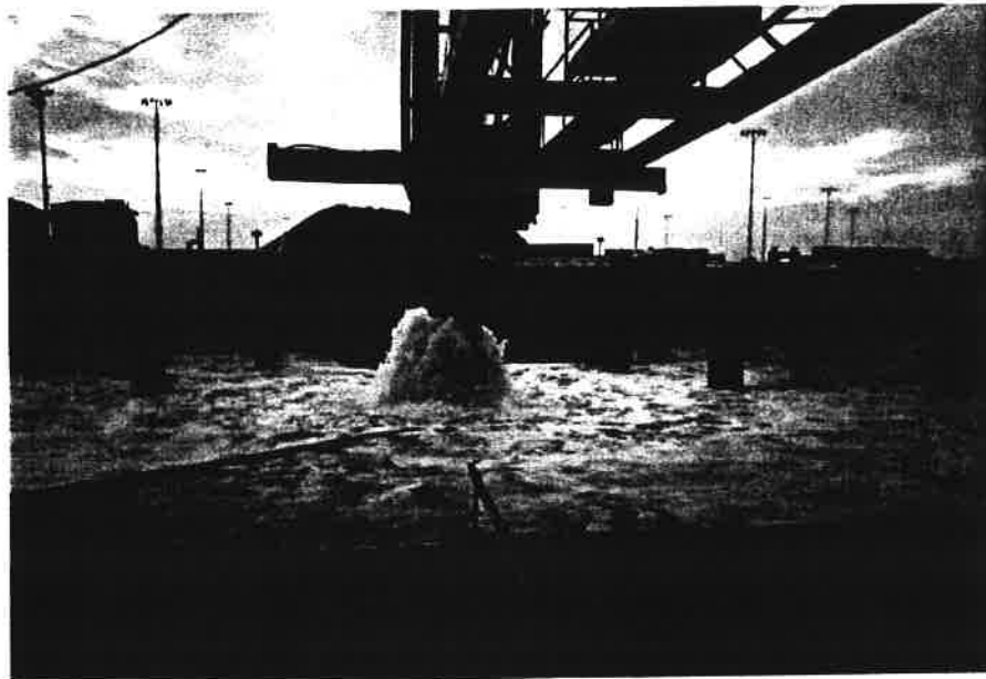
Figure 4. Driving of D Row Pile with PVC Shell Air Bubble Curtain System.
