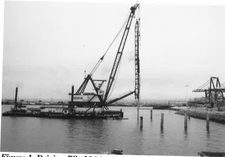
Figure 1. Driving Pile 284A.
