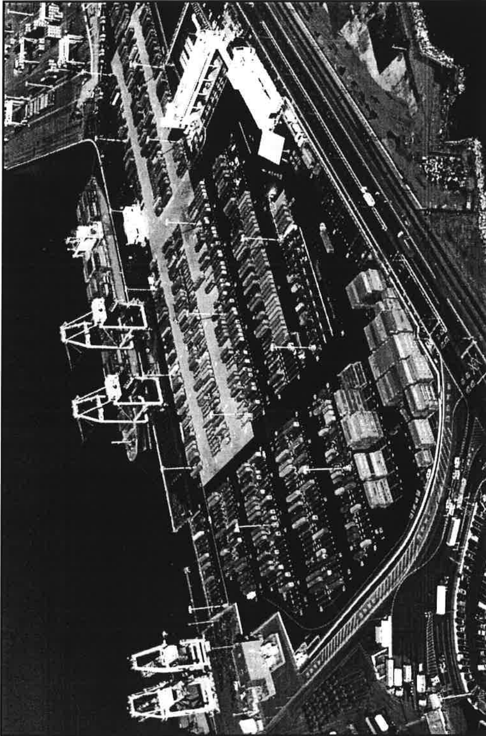
Typical Berth and Cranes
